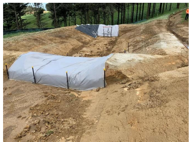
Figure 2. Sediment Retention Pond
