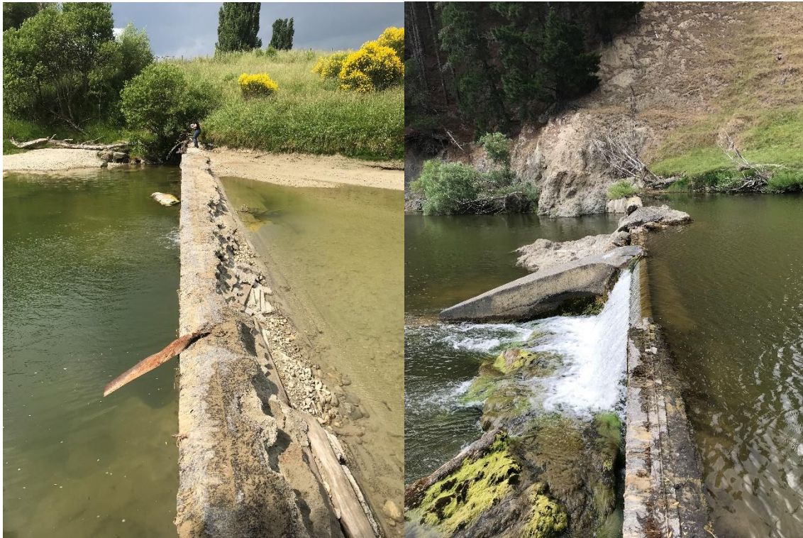
Figure 1: Akitio weirs – left, the rabbit weir (NB no water flows over the weir during low flows, only under it) and right, the salt water wedge weir.
