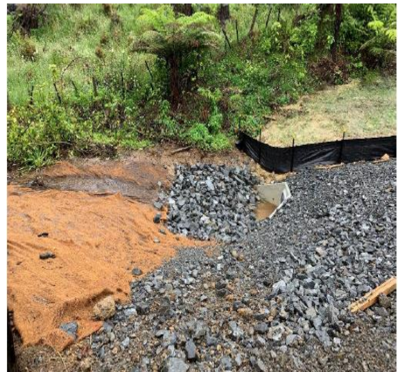
Figure 4. Culvert installation
