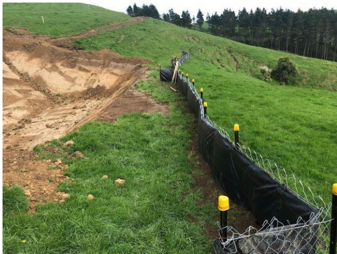
Figure 3. Super Silt Fence controlling sediment run-off while primary control is constructed
